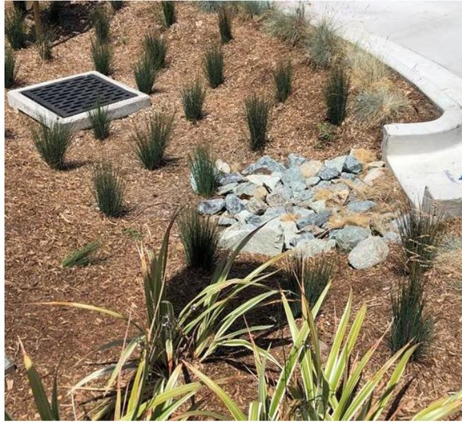
INFILTRATIVE BIORETENTION EXAMPLE
